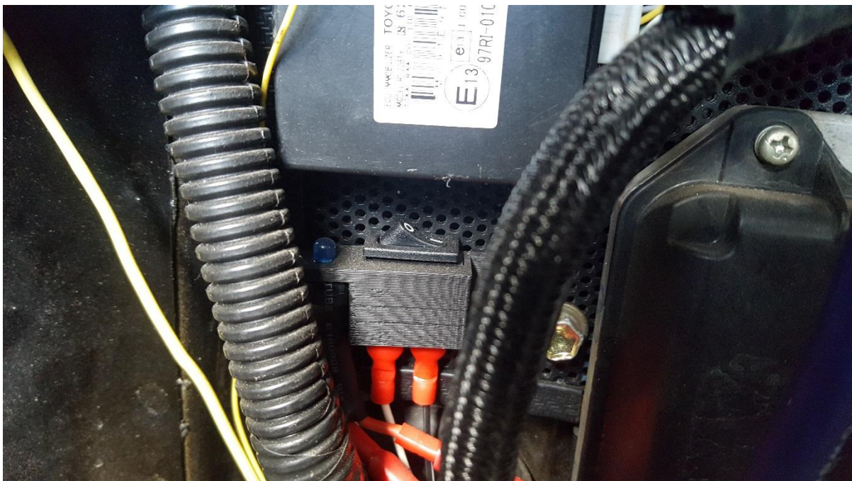
The photo below shows my key switch and security indicator LED
